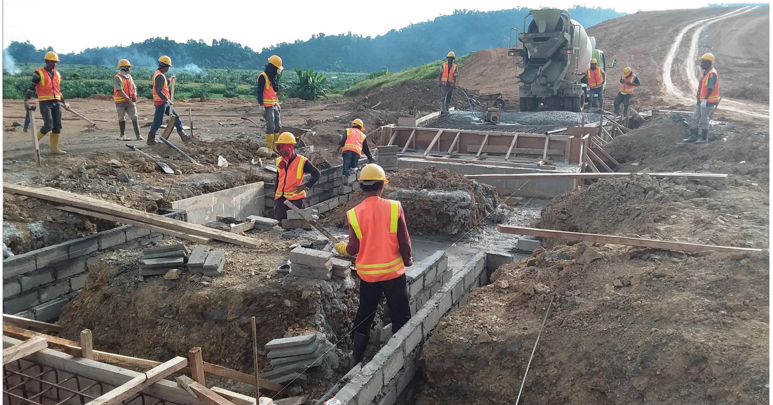
Oil Storage Tank Foundation
